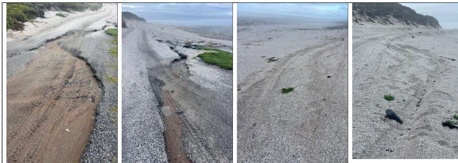
Figure 3: Photos of road provided by IAP
