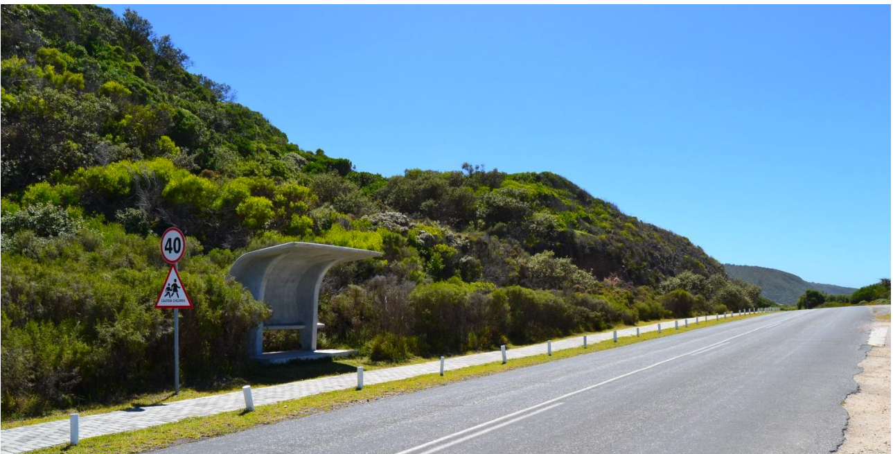
Figure 23: Photograph of the site taken from the parking area of the lookout point on the ocean side of the MR 394 scenic route. Note the steep cutting and density of vegetation covering the site (Smit, 2021)
