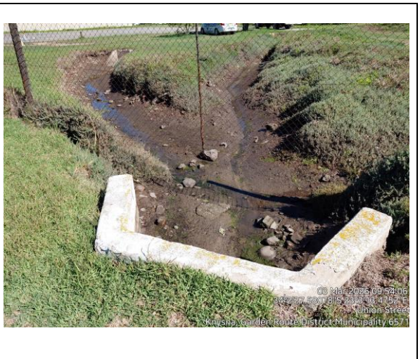
Fig. 8. A drainage channel runs through the testing ground and enters the estuary via a culvert.
