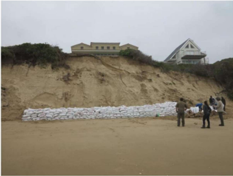
Figure 10.7. Emergency sand bags placed at Sedgfield (Myoli Beach) after a period of dune cliff storm erosion
