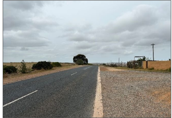
1b) Looking south-east along TR3302
