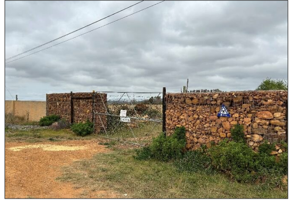
2d) Truck entrance directly east of residential access
