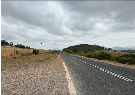
1a) Looking north-west along TR3302
