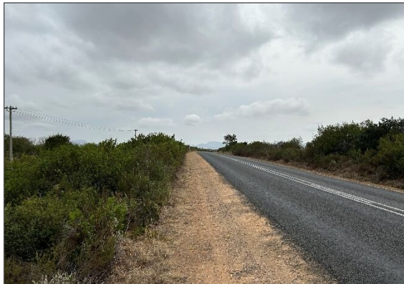
3a) Looking north-west along TR3302
