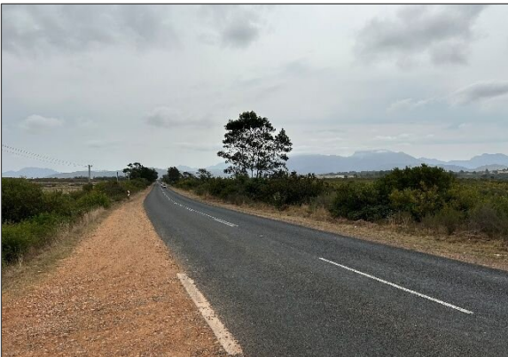
2a) Looking north-west along TR3302
