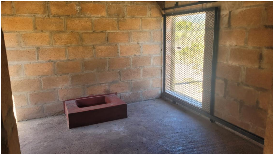
Example: Sliding Gates and Water trough inside Management Rooms, designed and constructed by J Olsen; Ubuntu Wildlife Sanctuary; Oudtshoorn
