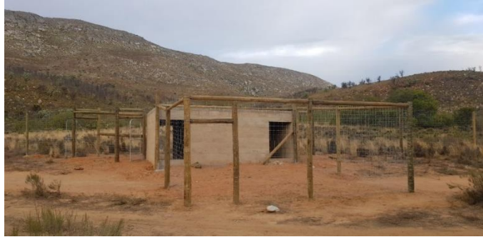
Example of Management rooms and camp (under construction), designed and constructed by J Olsen; Ubuntu Wildlife Sanctuary Oudtshoorn.
