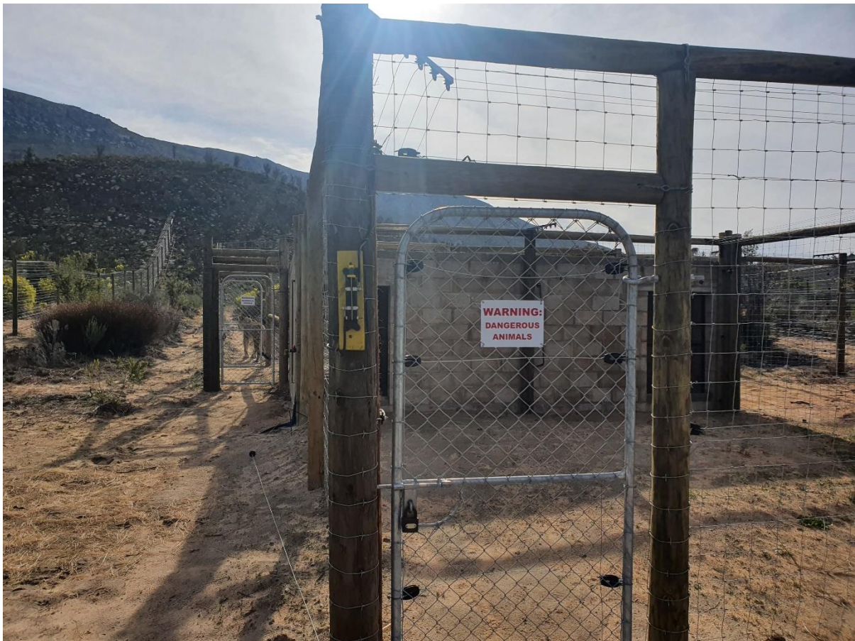
Example: Double gated access with warning signs and electric lines designed and constructed by J Olsen at Ubuntu Wildlife Sanctuary, Oudsthoorn
