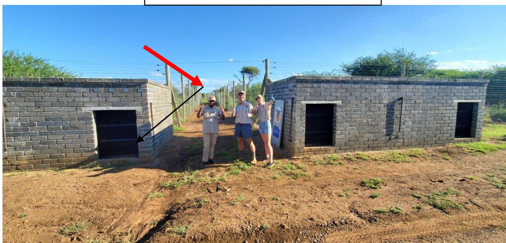
Example of two separate sets of management rooms, Limpopo Province. Note: Holding Camps are separated with a 3 m wide isle
