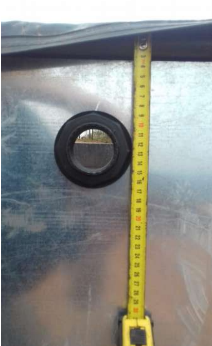
Picture Dam overflow 1 cm from top
