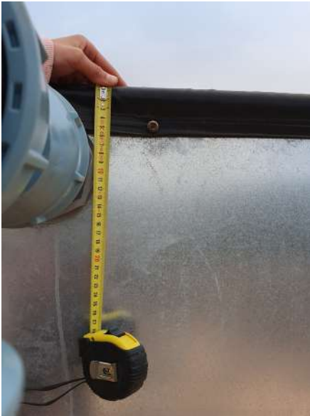
Picture 1 Dam 1 Overflow 1 cm from top
