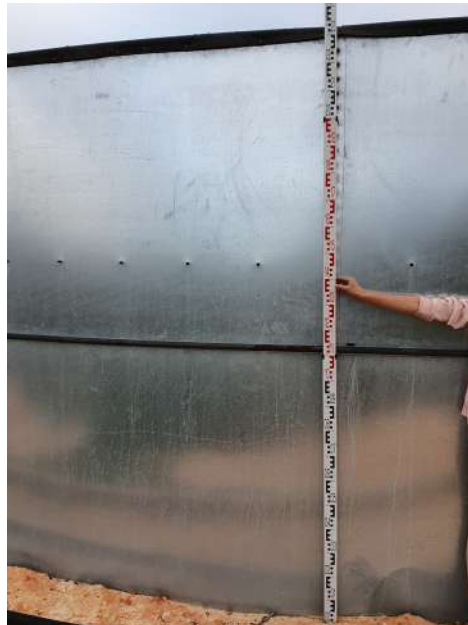
Picture Dam 1 height . m
