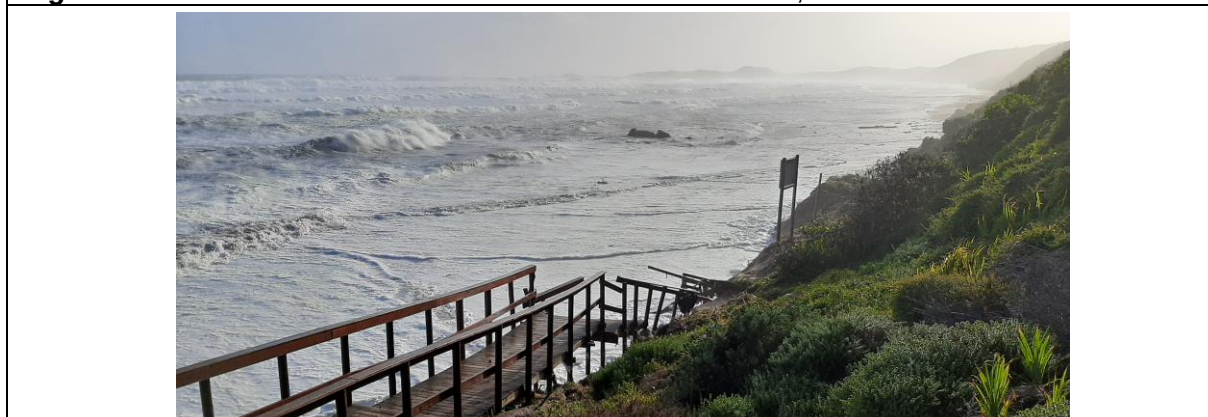
Fig.12. September 2023 storm surge, which washed away the Brenton on Sea beach walkway.
