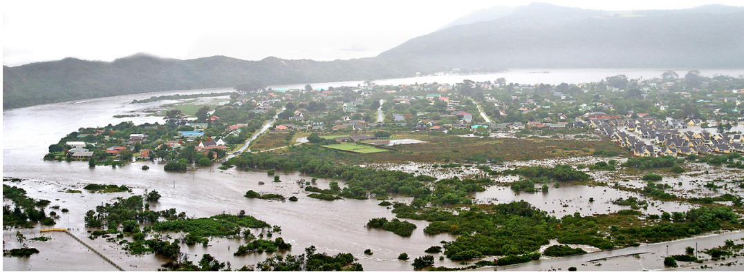
Photograph A2. November 2007: the area of the Group Housing north-west of bowling club is not flooded.
