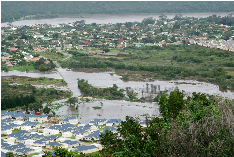
Photograph A1. August 2006: the Perdespruit causeway backs up water upstream to Montage Village and erf RE1627 . The area of the Group Housing area is not flooded
