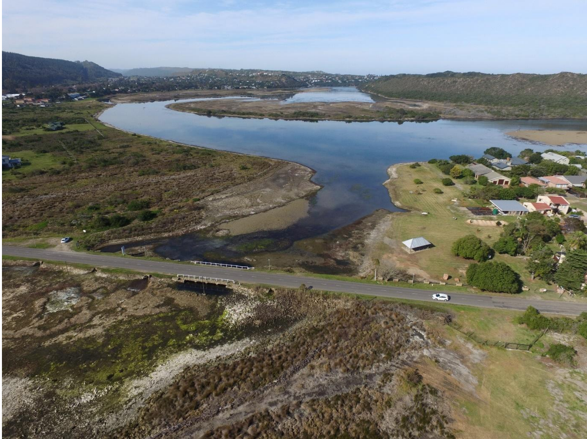
Figure 13. Flow restriction point at Dr Malan Street crossing. Note the difference in sedimentation upstream compared to downstream of the bridge.
