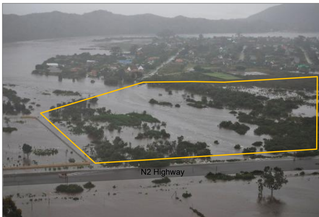
Figure 8. Photo of part of Sedgfield during flooding in 2007. View looking south shows the N2 Highway and the general area of RE/1627 (yellow area).
