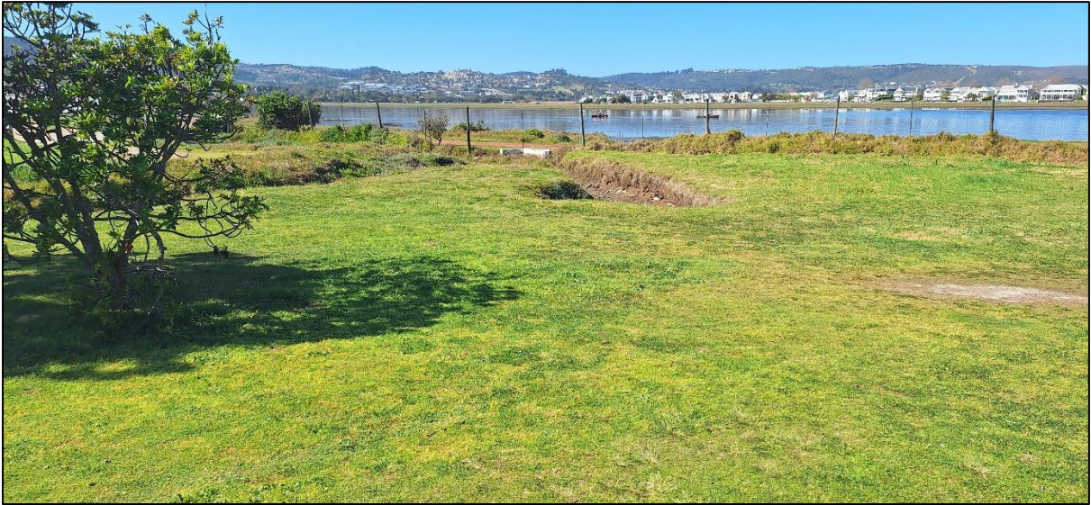
Plate 3: A photograph taken of the three stormwater drains on the property but adjacent to the site
