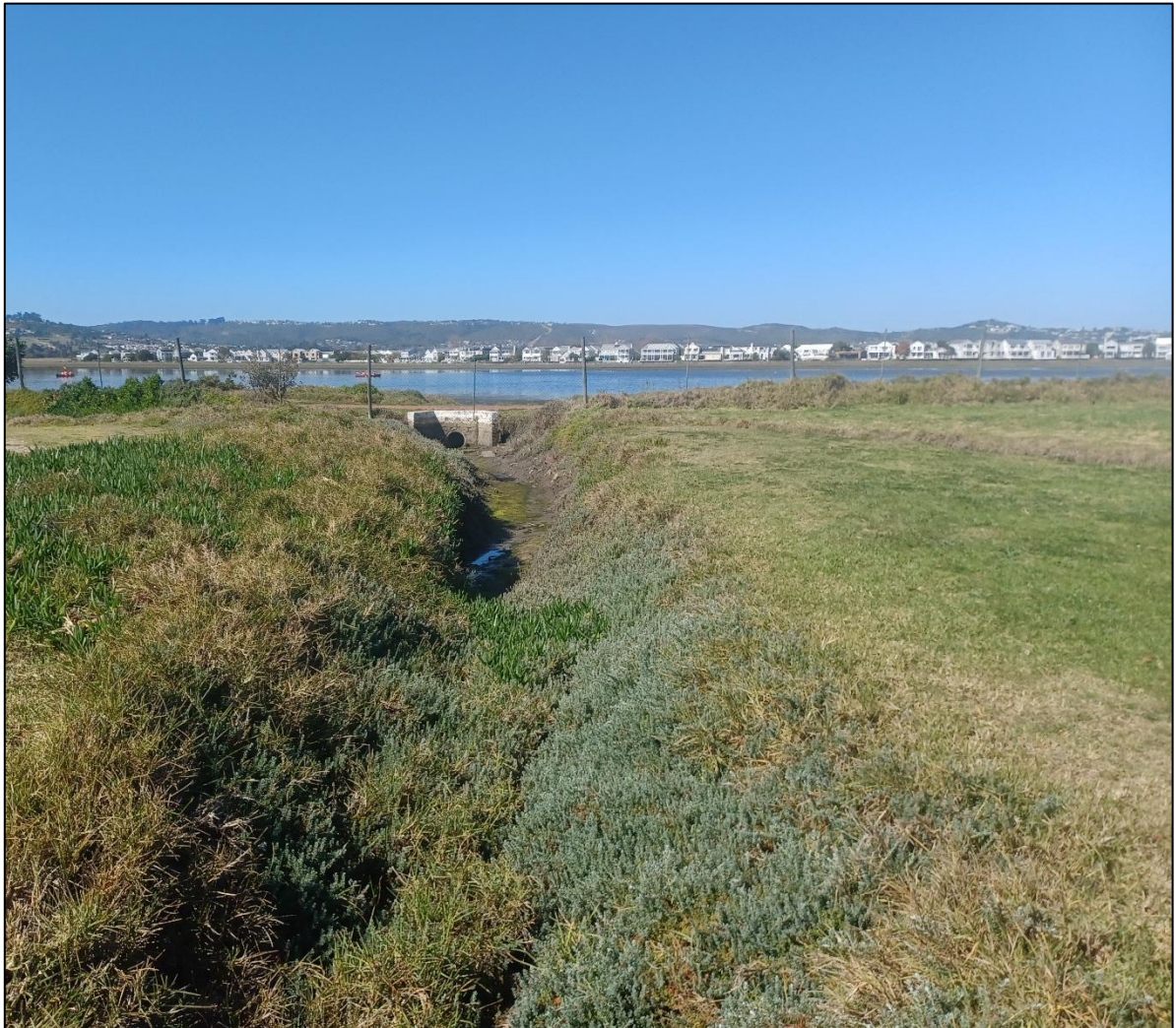
Plate 4: A photograph taken of one of the drains showing active saltmarsh area where the drain is below the HWM, note the left bank where the vegetation is not mowed.
