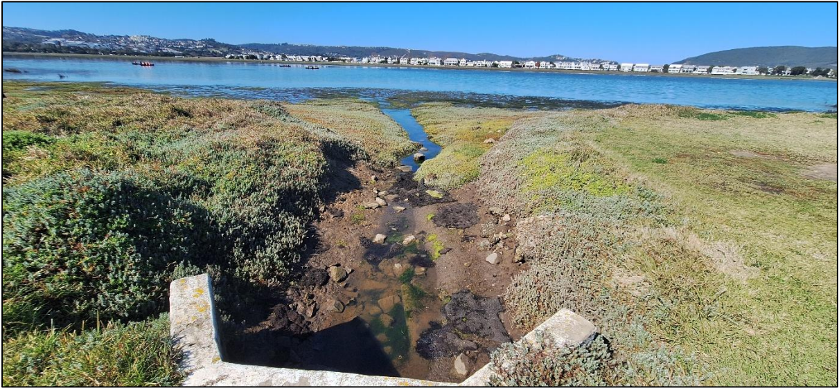
Plate 7: A photograph taken of the drains discharge point showing active saltmarsh area and base level of the estuary.
