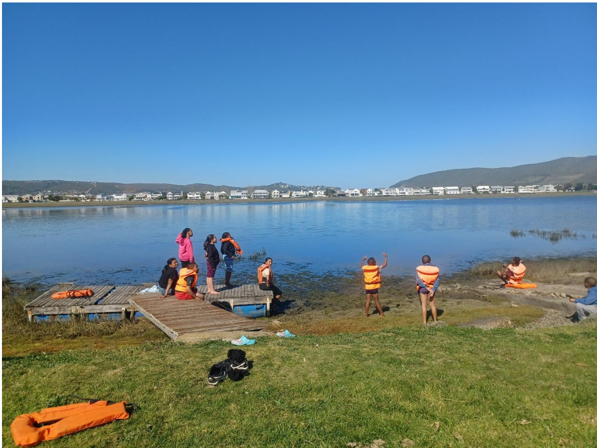
Plate 3: A photograph of the Jetty and slipway that the South African Sea Corp facility uses which will require maintenance and like for like replacement in future
