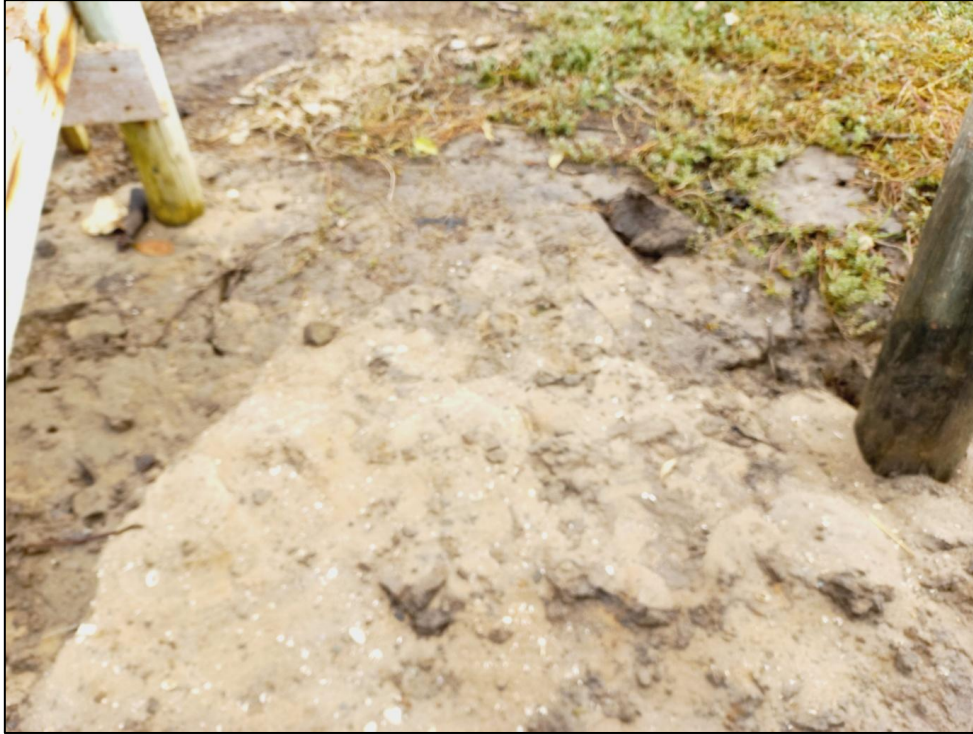
Figure 9: Photograph showing an example of the localised changes to salt marsh from excavations for jetty construction
