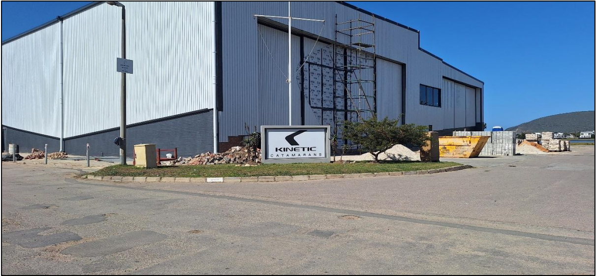
Plate 1: Photograph taken of the existing facility located adjacent to the site
