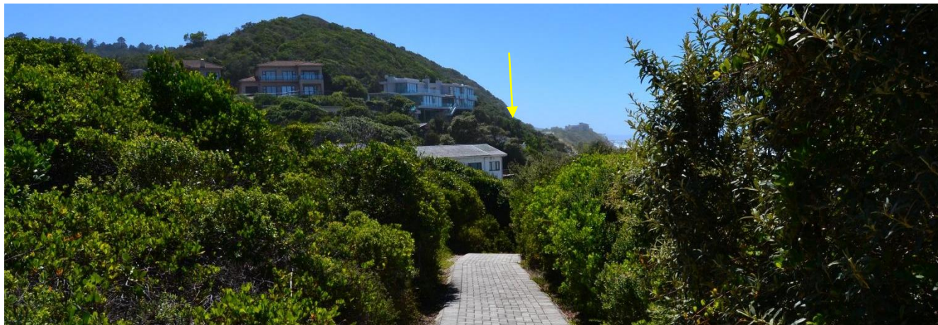
Figure 56: Site photograph taken from the elevated pedestrian walkway alongside the MR394 scenic route at 500m from the project site, looking east (Smit, 2021)
