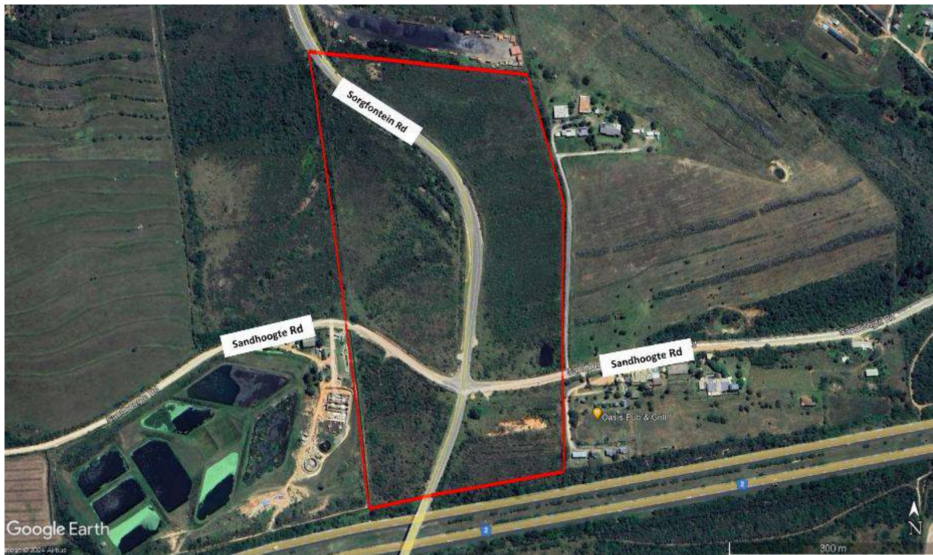
Figure 1.2: Aerial image of Erf 139.
