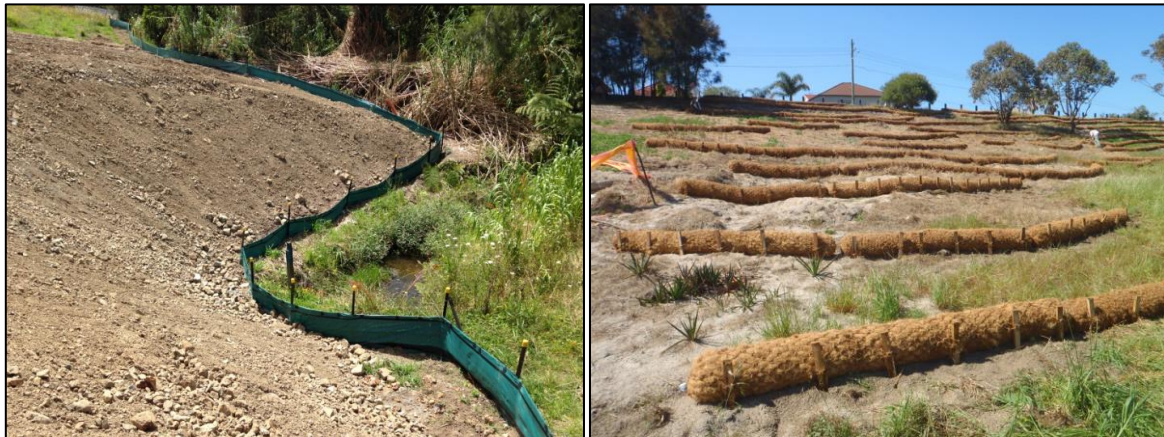
Figure 20: Examples of silt fences (left) and coir logs (right) used to trap sediment mobilised from steep slopes.
