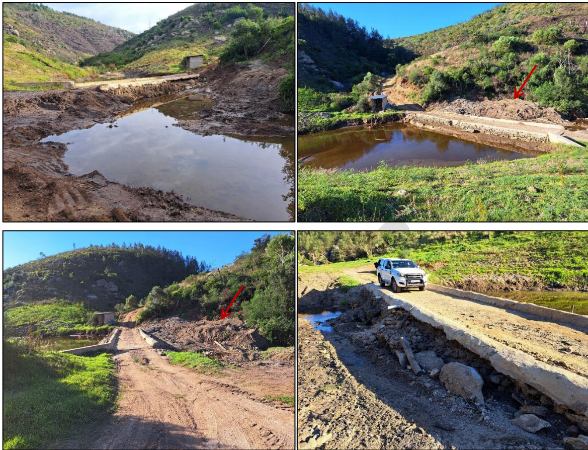
Figure 14: Photographs of the road crossing and small instream dam upstream of the road (red arrows indicating sediment dumped in the channel of the Ruiterbos River).
