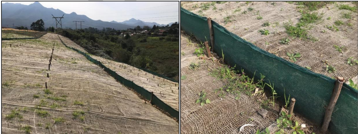
Figure 15: Images of installed soil saver matting and silt fences several weeks after installation
