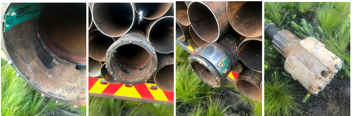
Plate 2 – Indicates the setup of the ODEX drilling technique equipment.
