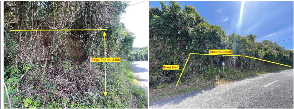
Figure 38: Southern boundary of the property showing edge fall onto Waterside Ride
