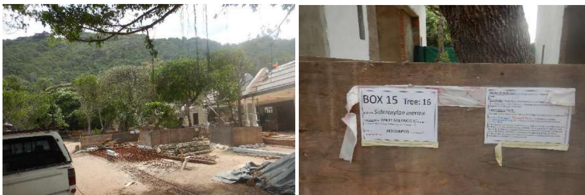
Figure 19: Images of a construction site where protected and indigenous trees were marked and protected on the site.
