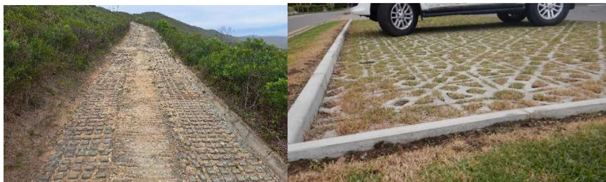
Figure 18: Examples of Open pavers and permeable road surfaces. The image on the left shows a minimal edge effect along the site of the road, where natural fynbos vegetation grows directly adjacent to the road.
