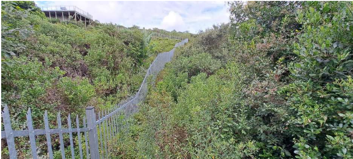
Figure 21: An example of a palisade fence that would allow for the movement of small animals and seed dispersal with no associated fire break along the fenceline.
