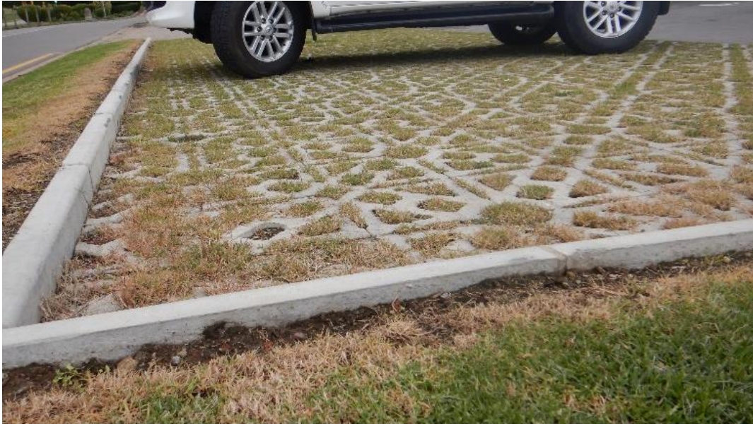
Figure 20: A local example of the use of open pavers for car parking in George.
