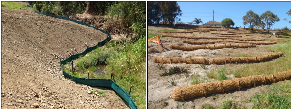
Figure 10: Examples of silt fences (left) and coir logs (right) used to trap sediment mobilised from steep slopes.
