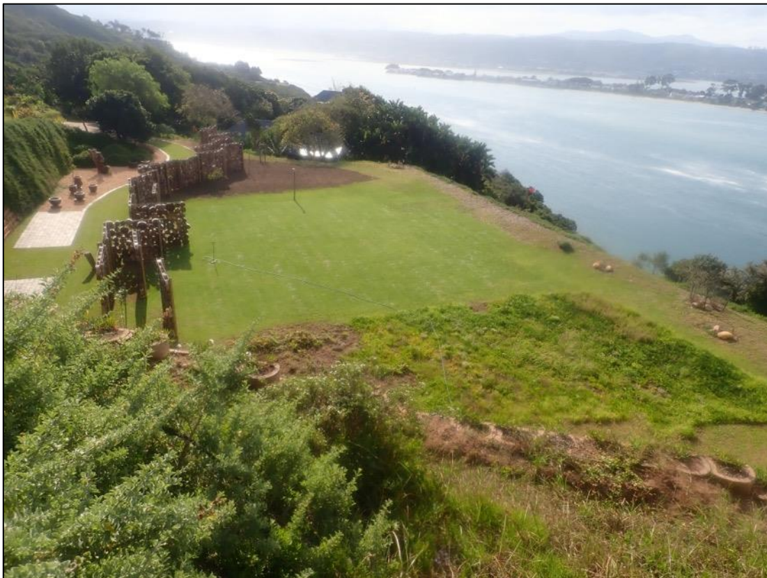
Figure 19. The Highly degraded landscaped habitat can be seen in the top of the image with an open grassy area and some remnant Highly degraded vegetation at the bottom of the retaining wall. Some Degraded Dune Thicket can be seen in the foreground
