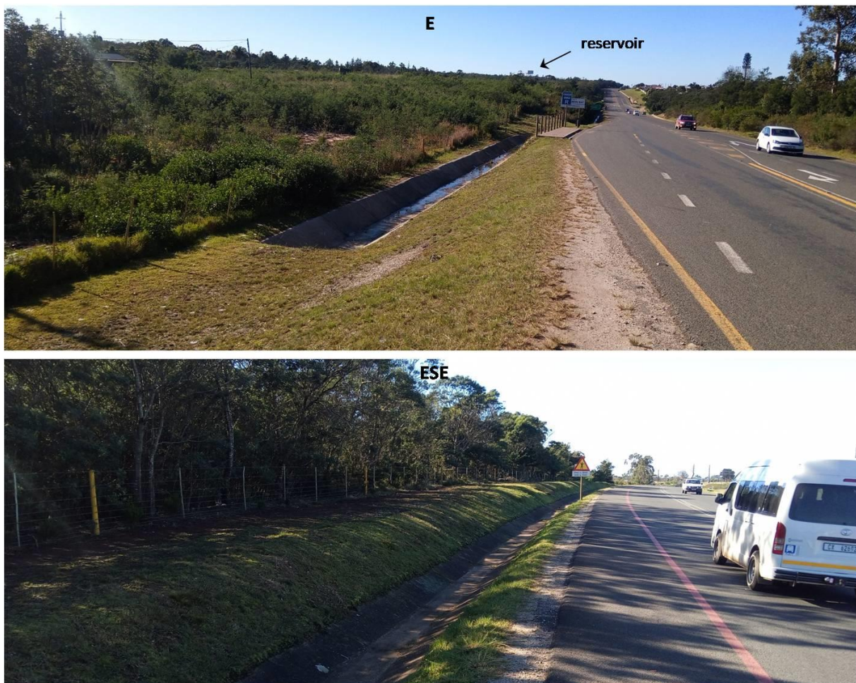
Figure 5. Views towards the study area from the N2. 33/437 is to the left of the reservoir (top) and set back some 90 m from the tree line adjacent to and north of the N2 (bottom).
