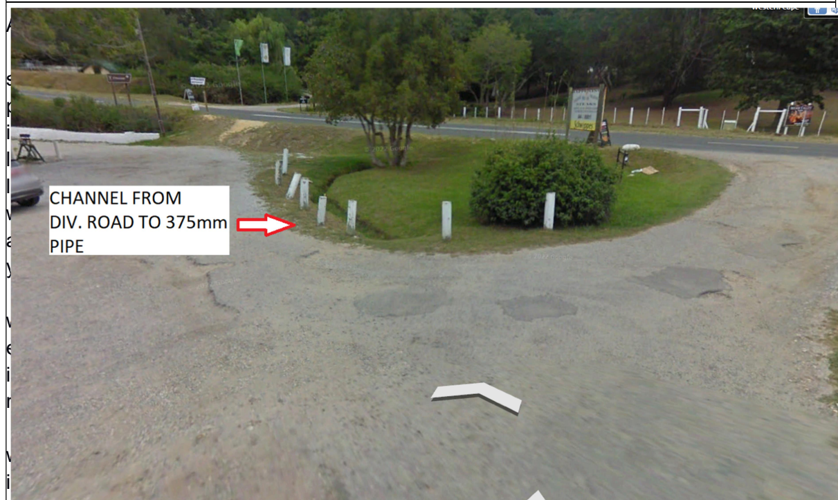
FIGURE 7: CHANNEL LEADING TO EXISTING 375MM PIPE
