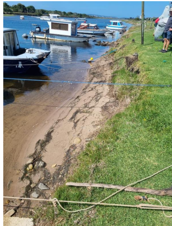
Figures 5 & 6: Erosion of embankment is evident with a dominance of grass cover.
