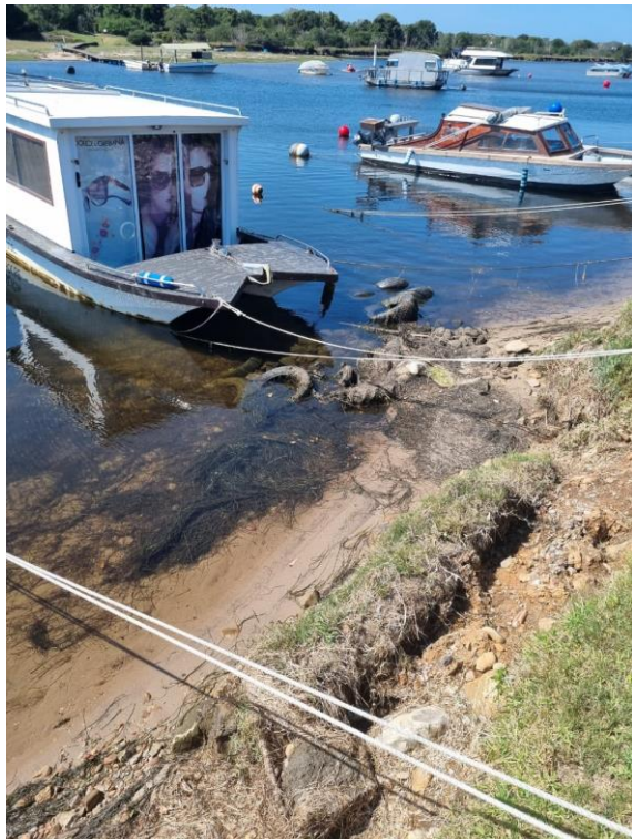
Figures 5 & 6: Erosion of embankment is evident with a dominance of grass cover.
