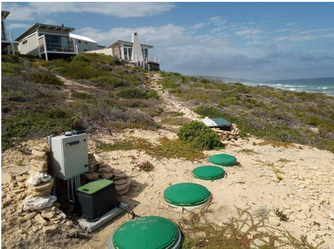
Fusion installation at De Hoop Nature reserve
