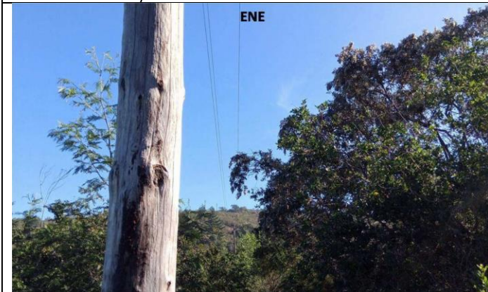
20. The overhead power line crossing Erf 1058 (Dr. Peter Nilssen).
