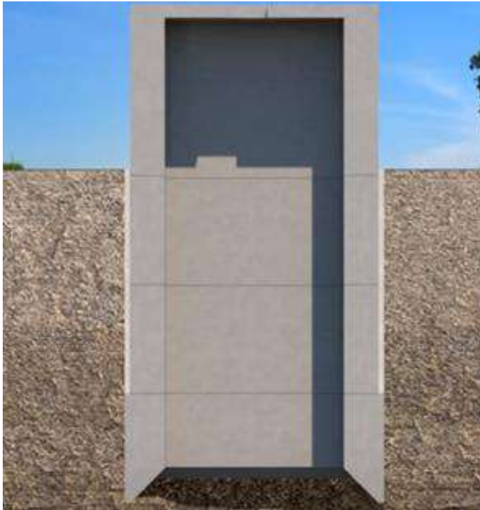
Figure 4-5: Placing of more Concrete rings
