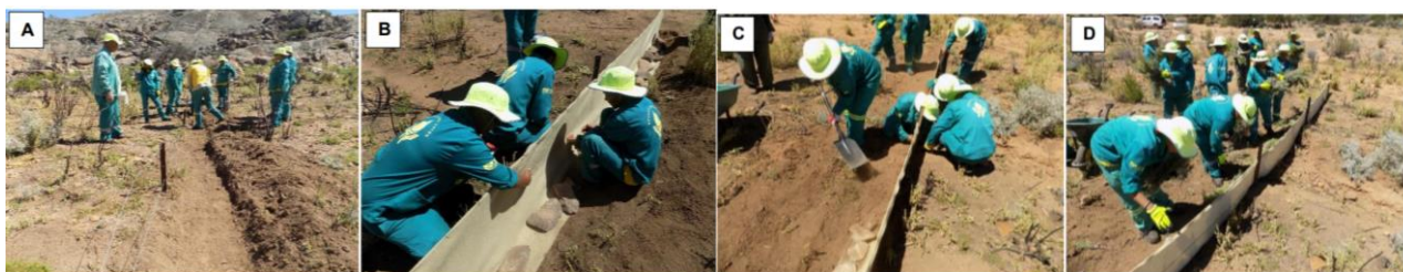
Figure 12: Installation of the soil erosion control fence. A: Installing the standards and wires and preparing the trench. B: Fitting the geotextile, tying it on with wire. C: Filling in the trench over the geotextile. D: Applying a mulch against the completed fence (Photos courtesy Ken Coetzee).
