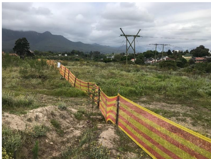
Figure 7. Example of temporary fencing of a riparian buffer zone during the construction phase.
