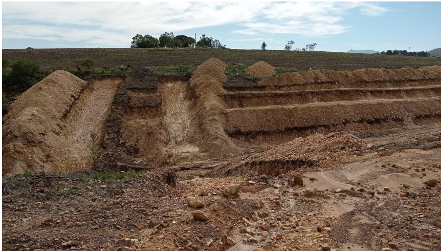
Figure 5: Stockpiled fill material
