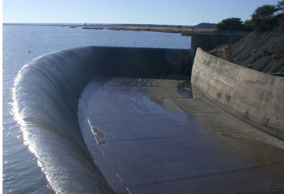
Figure 8: Side-channel spillway example
