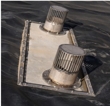
Figure 10: Typical submerged inlet (two pipes)
