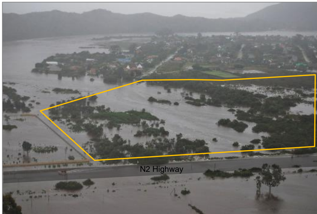
Figure 2. Photo of part of Sedgfield during flooding in 2007. View looking south shows the N2 Highway and the general area of RE/1627 (yellow area).
