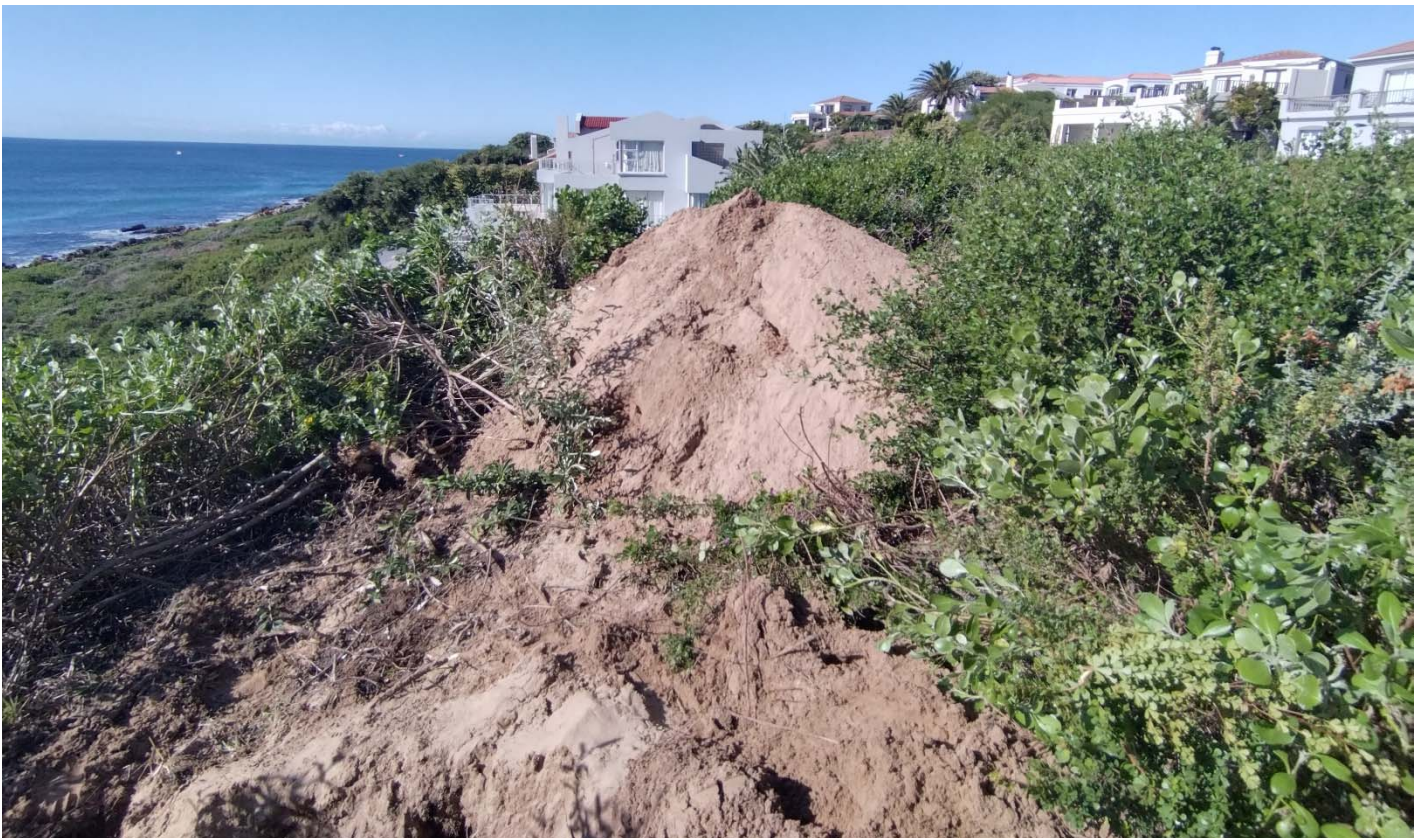
Figure 2: Photo of sandy soil excavated from test pit TP1
