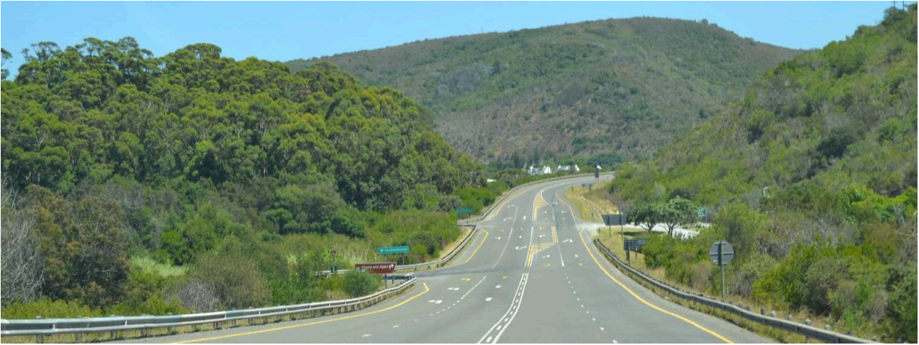
Figure 12: Site photograph of the N2 freeway just before the Keurboomstrand access road turnoff (left), demonstrating the typical inland topography and vegetation cover (Smit, 2021)
