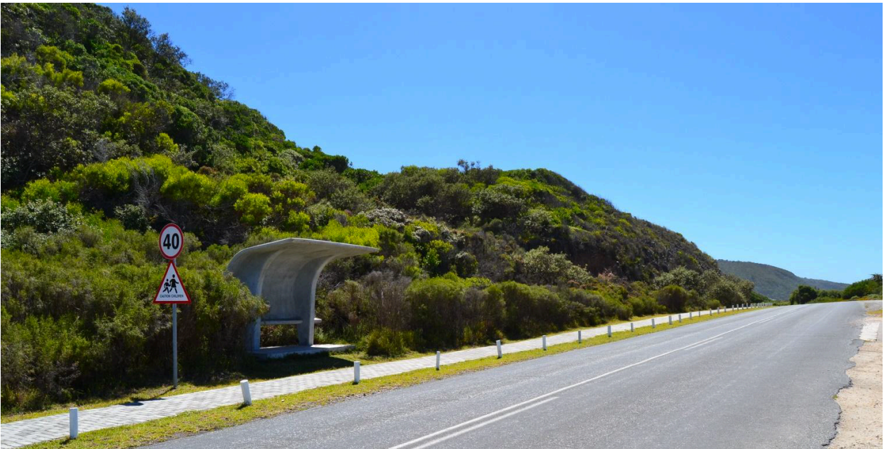
Figure 23: Photograph of the site taken from the parking area of the lookout point on the ocean side of the MR 394 scenic route. Note the steep cutting and density of vegetation covering the site (Smit, 2021)
