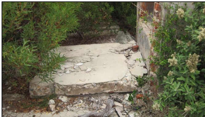
Plate 18: A concrete platform in front of the hearth. Grooves for wood panels can be seen in the edges of the slabs behind. Plate 19: The brick hearth and chimney is of a vernacular style although layout of the slabs does not suggest a vernacular shape.
