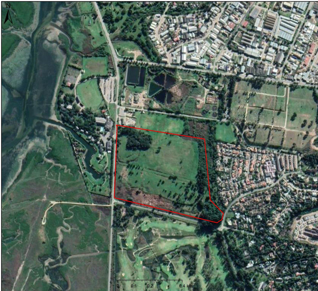
Site and surrounding Areas
