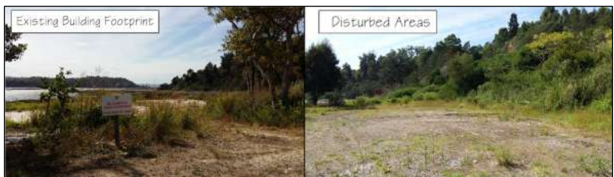
FIGURE 6: EXISTING FOUNDATION OF REMOVED STRUCTURES ON SITE
