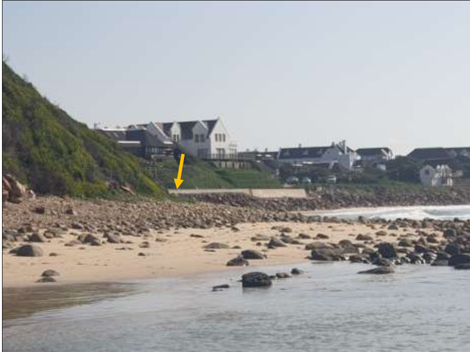
This photograph shows a close-up of the middle section of the proposed boardwalk 34°10'11.49"S 24°50'1.23"E. The concrete retaining wall can be seen in the distance (start of retaining wall – orange arrow).
