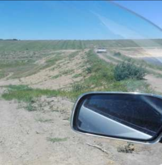
5. Area of reconstructed dam wall
