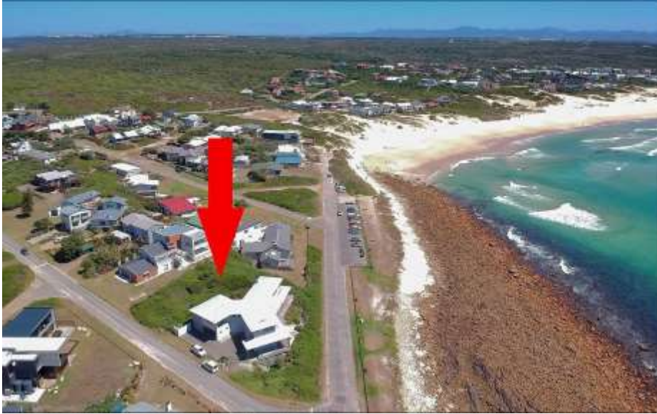
Aerial view of Erf 23
